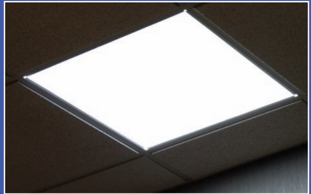
This 23.5" x 23.5" troffer downlight features a slim, lightweight backlight assembly that is edge lit with high efficiency LEDs that focus the light into a high-performance light guide.
